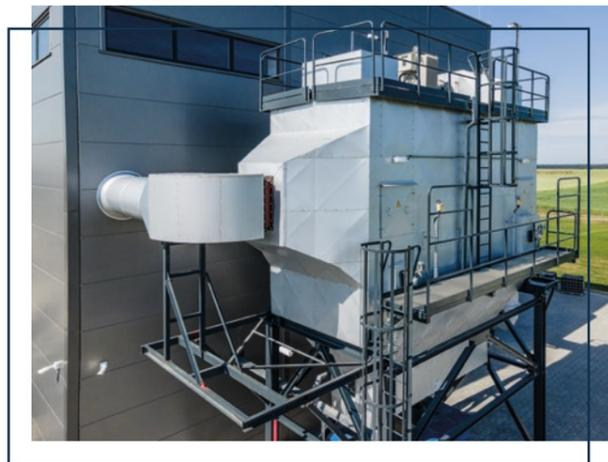
Electrostatic precipitators for solid fuel boilers are also a very effective way to reduce harmful emissions into the atmosphere. Electrostatic precipitators use the electrostatic phenomenon to separate particulate matter from the flowing air.
