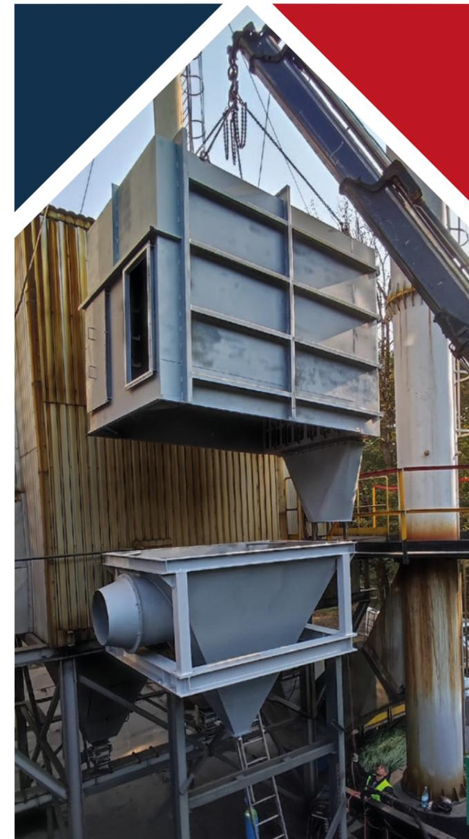
Modular horizontal bag filters are state-of-the-art devices for efficient industrial dust gas purification, combining high filtration efficiency with optimal operating and investment costs. Their applications span a wide range of industries — from power generation and metallurgy to the chemical, food and cement industries. With ATEX versions, they also enable dust removal from explosive dust-air mixtures.
